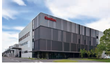
Shiga Plant (Power supplies)
